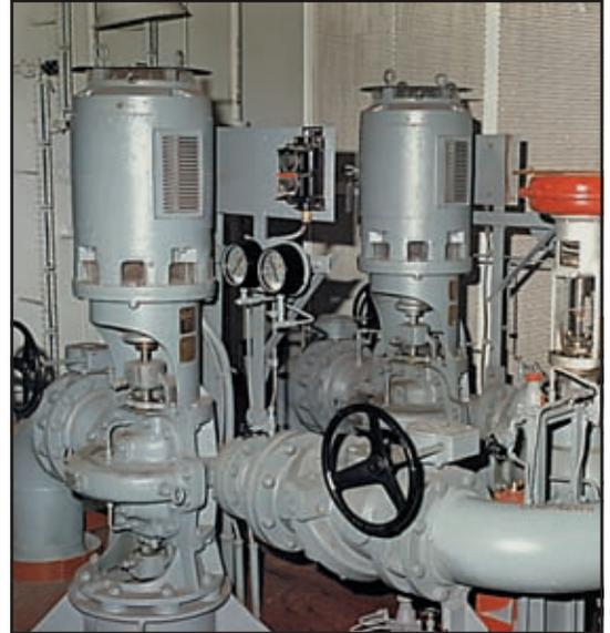
The pumps of this fresh water circulation system are powered by our 50-HP, 1800-RPM vertical P-base motors.
