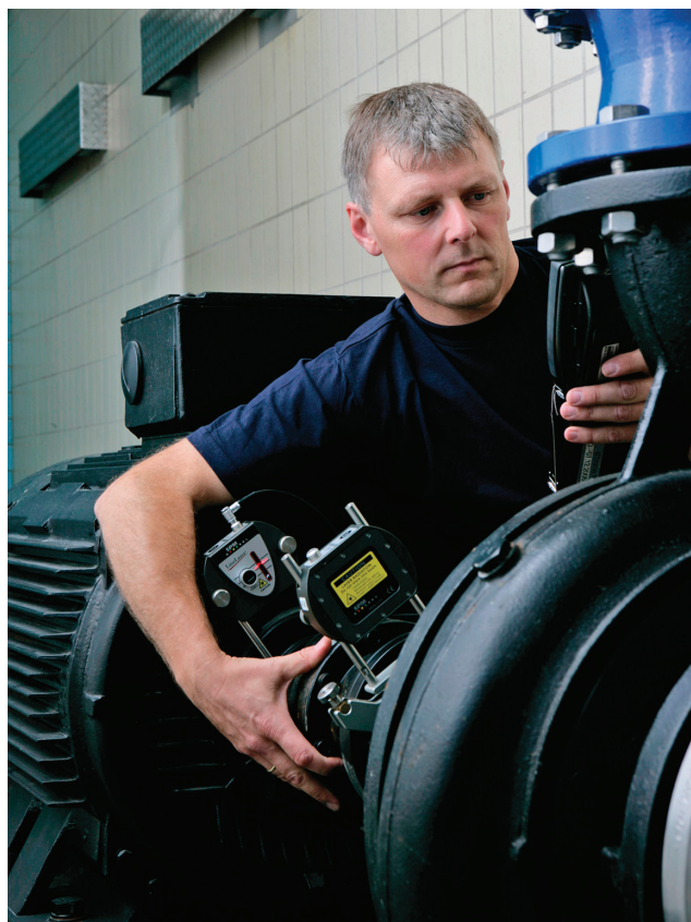
Alignment labor for an end-suction frame-mounted pumps can be time-consuming and costly.
