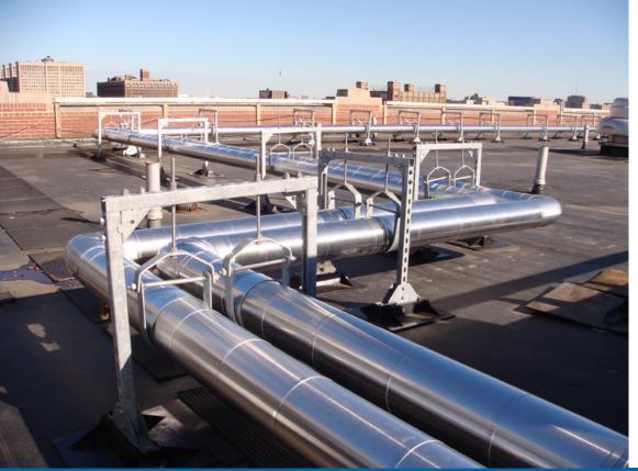
For conduit and other small electrical piping. Uses channel strut to allow for the addition of pipe clamps, and ranges in height from 2.5" to 18", and in widths up to 48".
