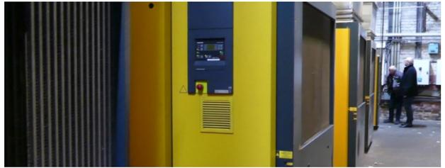
Second, let's look at an industrial signage production facility where we installed a 1.2 MW compressed air system. Heat recovery uses heat exchangers installed on the tops of the compressors. This configuration was preferred to take advantage of the available space. The total recovered energy is around 800 kW for the complete system. It is reused in the customer's heating system."
