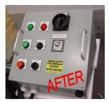
The older technologies used in the original panel required multiple individual components with additional wiring, all of which creates additional opportunities for the panel to fail. Both panels got the job done although the new panel provides additional features and much tighter control with fewer components and significantly reducing the MTBF (Mean Time Between Failure).
