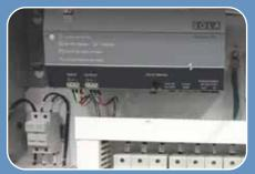
**OPTIONAL BACK UP POWER SUPPLY** Allows default positioning and controlled switching on power failure.
