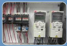
VARIABLE FREQUENCY DRIVES Enhances pump performance and saves energy. Output pump pressure (PSI) is set on touch screen.
