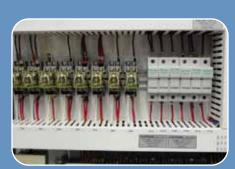
ISOLATION RELAYS Protect the PLC from damage on device power up surges and faults.
